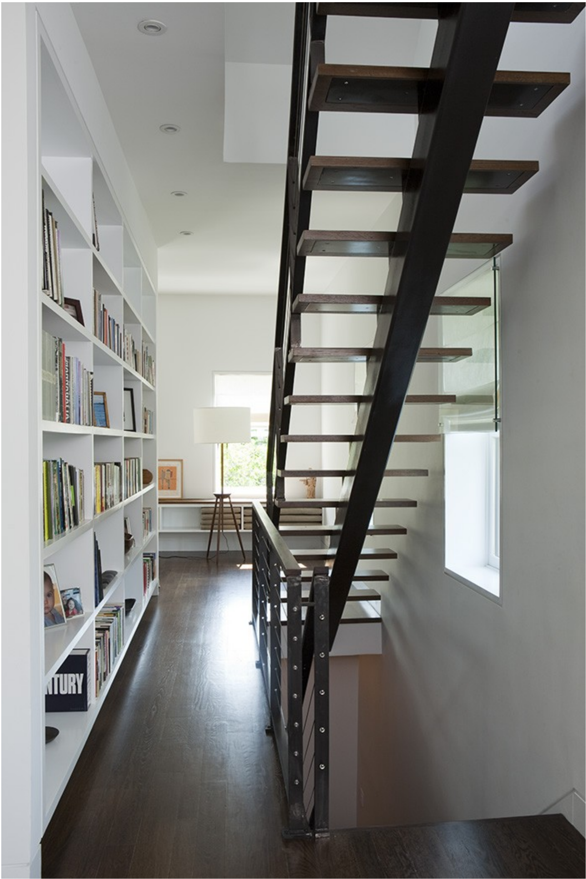
Above: Detailed as a floating object, the stair leads to the rooftop garden. The architects animated the stair wall by slotting a bookshelf into it.
